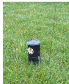
Figure 6. Clogged nozzle.
