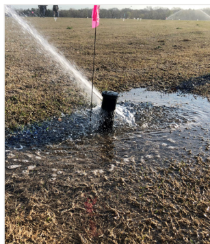
Figure 5. Broken sprinkler.
