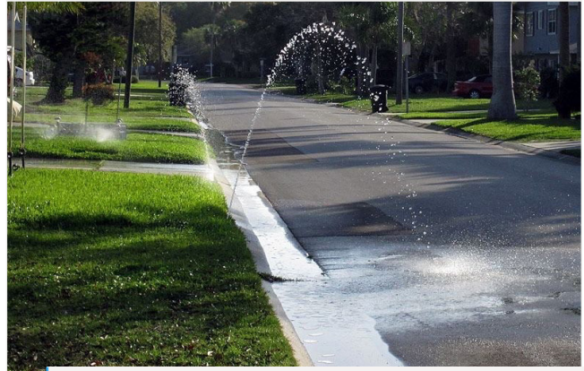
Figure 5b. Runoff caused by a misaligned rotor sprinkler
